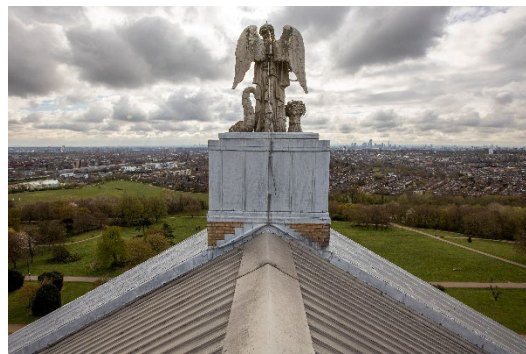
Wire in the Sky, ongoing
